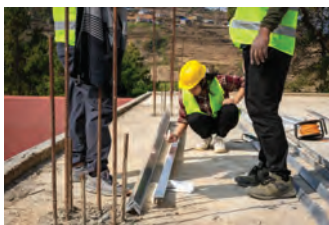
Measurements being taken for the construction of trusses
