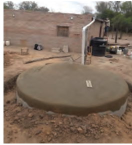
Water storage facility under construction at a residence
